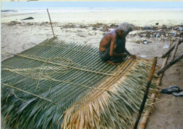
Making roof from rattan and nipa palm
